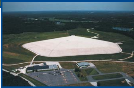
Weldon Spring Disposal Cell, 2002
